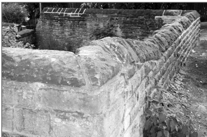
STRUCTURE: The stone pinfold at the bottom of Headlands Road
